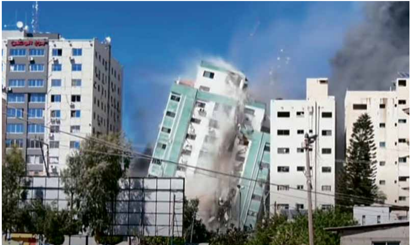
A residential tower block in Gaza City is flattened by Israeli bombs - an unstated form of 'collective punishment' inflicted on the Palestinian population
