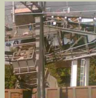
The collapsed waste hopper
